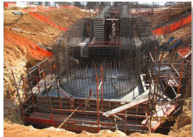
Construction of a sludge recycling pump station
